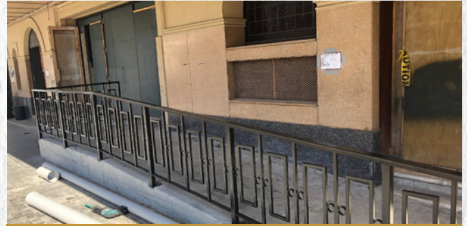
The new Hawke's Bay Opera House accessibility ramp and balustrade.
